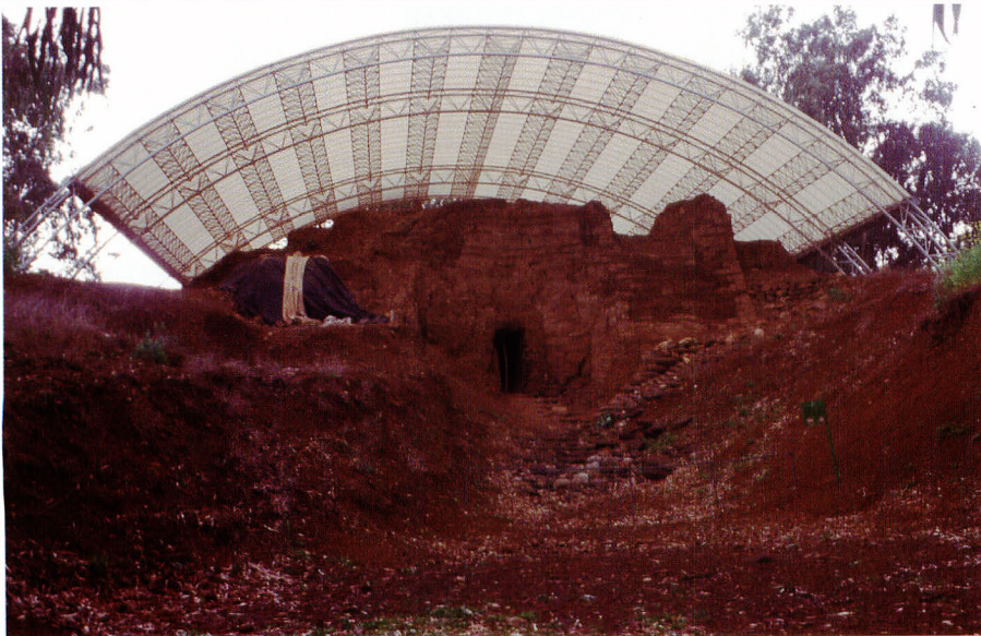
c: View of the eastern façade of XVIII th Century B.C. (Middle Bronze Age) gate of the Canaanite city of Laish at Tel Dan, northern Israel. This famous triple arched gate in unbaked bricks of Tel Dan (built in three radial courses) the span of which is about 2.30 m, has been excavated by Professor, archaeologist, Avraham Biran. It is part of a defence system which consisted of sloping ramparts and glacis. Stone constructions have been found, built against and close to the mud structures whose successive layers are made with brown and grey coloured bricks.
