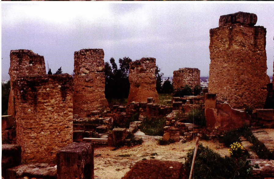
c: Detailed view of the columns in "pisé" erected by the Roman, when, some years after the destruction of Carthage, they have refilled the slopes of the hill of Byrsa for levelling a new platform which will bear the new Forum and Basilica of the Roman Carthage (1 st Century A.D.). This structural performance consisting in building earthen columns for realising new footings is in fact common in the Roman engineering practices. Other similar traditions are existing in the history as this can be observed at Susa, Khuzistan, on the Darius' Palace.
