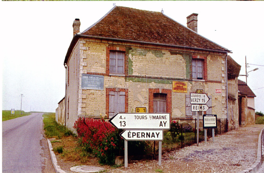
b: Still in Champagne, near the cities of Ay and Epernay, well known for their excellent vineyards, numerous villages and rural houses are built in unbaked earthen blocks locally called “carreaux de terre”. This tradition is notably visible in villages located along the Marne River Valley but is not still living.
