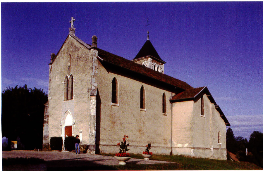
c: A rare and nice example of a Christian church built in “ pisé ”, plastered with a thin lime distemper, in Isere, village of Charancieu located around 30 km north Grenoble. This church has been built at the middle of the XIX th Century. All walls, excepted those of the bell tower are in “ pisé ”.
