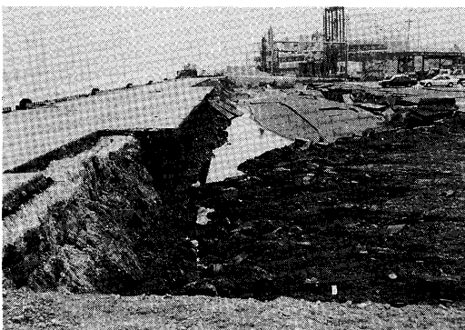
Photo 14 The soil failure at Portpier, Kobe City, caused by liquefaction (b).
