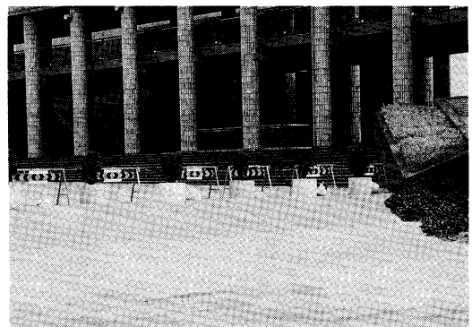
Photo 16 The settlement at Portpier. The ground subsided up to about 1 m.
