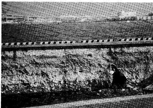
Photo 13 The soil failure at Portpier, Kobe City, caused by liquefaction (a).
